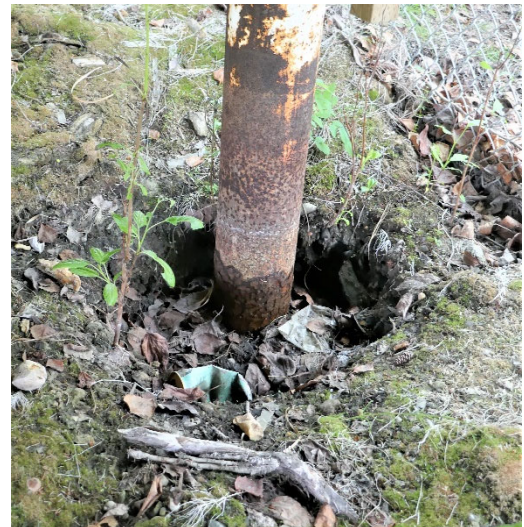
Figure 3: Depression Around Thermo Ring-Pile
