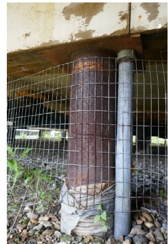
Figure 5: Frost Jacking Thermistor Tube
