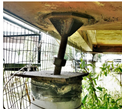
Figure 6: Failing Adjustable Pile Cap
