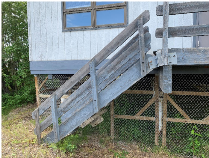
Figure 2: Distressed Stairs at East End of Dental Clinic
