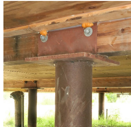
Figure 4: Original Main Clinic Pile Cap
