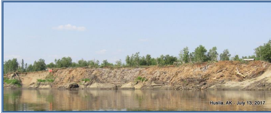
Figure 4-9 Cut Wood Debris Used to Armor Embankment
